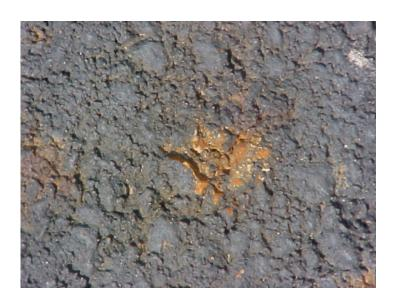
begin to appear as silvery streaks on the sealcoated surface. As more time passes, these streaks turn brown and finally the rust spots erupt through the sealcoating.
